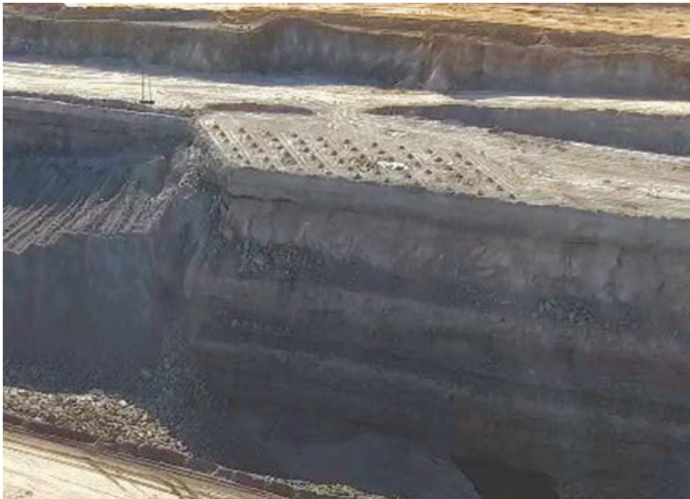
An Indiana mine uses Dyno42 and SignaShot to reverse a costly decision to deck blasts. The software systems mandate use of electronic detonators, which provide the required timing accuracy. (Photo: Dyno Nobel)
